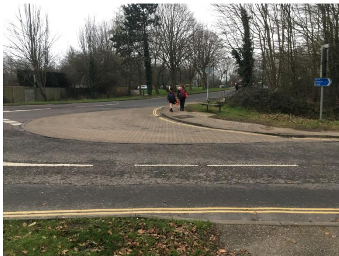
Photo 5: Existing overrun area
